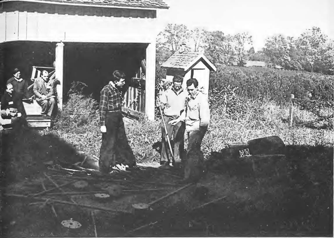
The Construction Situation
