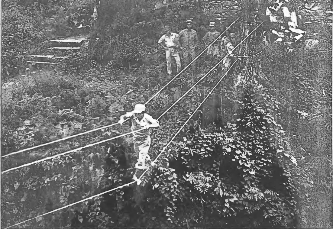
The Bridge Construction Situation at H
