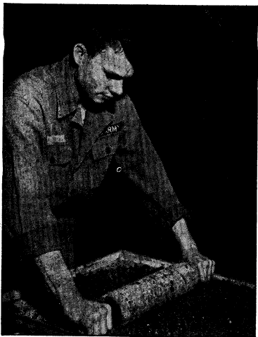
MUD PIES —Rolling them out is Private John C. Stinson of Ordan, Utah. The dirt is used in tests at the Army Engineer Soils Laboratory, Fort Leonard Wood, Mo., to determine its compactability. Each tests tell which soil meets Army standards for use as base for roads, airplane runways, highways, or dirt-fill dams.
