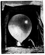
HOLDING THE BAG!-This helium-filled balloon soon will be on its way up into the stratosphere to gather valuable weather data for Army anti-aircraft sharpshooters at Camp Nupunja, Okinawa. Balloons like this haul aloft radiosondes—electronic weathermen which relay back to earth weather data vital to pin-point accuracy. PATRONIZE THOSE ADVERTISERS WHO HELP MAKE THIS PAPER POSSIBLE
