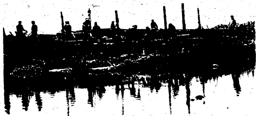
Men of the 77th Combat Eng Bn, 25th US Inf Div, erect foundation for bridge to be constructed across the NADAE-C.O. River, southeast of PUMHANG, Korea.
