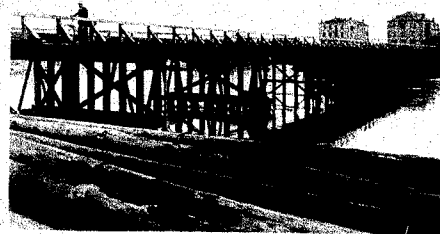
POMPEY BRIDGE OPENED TO TRAFFIC 8 NOVEMBER. WITHSTOOD ALL HEAVY FLOODS
