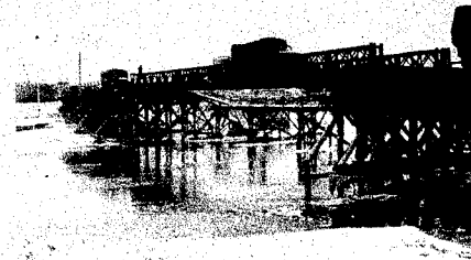
BRIDGE OVER THE SEMOIS RIVER AT FLORENVILLE
