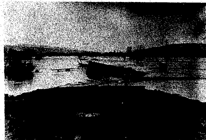
VANDIERES BRIDGE AFTER FLOOD HAD COVERED APPROACHES AND BAILEY BRIDGE HAD BEEN PULLED BACK TO SAVE IT FROM DAMAGE
