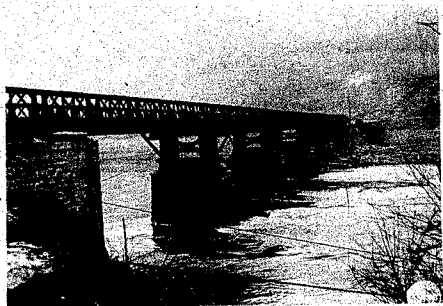
270-Foot Bailey Bridge Across Sure River at Echternach
