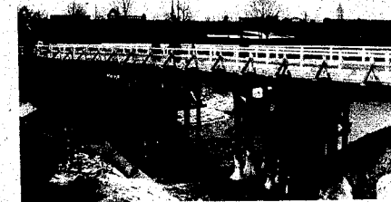
PILE BENT BRIDGE OVER SELLE RIVER IN METZ
