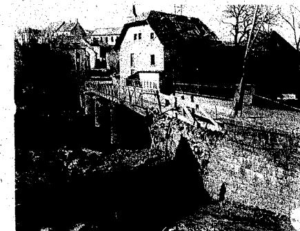
Bridge Across Nims River at Rittersdorf
