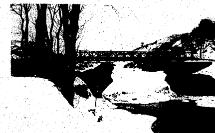
Seventy Foot Double-Single Bailey Bridge at Lutzhausen
