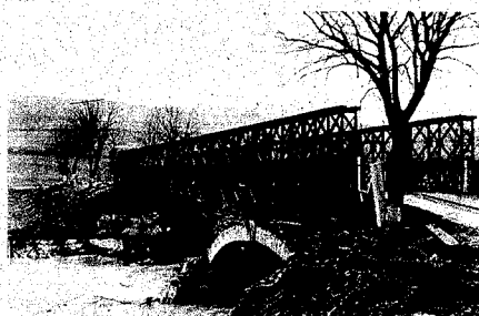
Bailey Bridge Across Our River at Oberhausen
