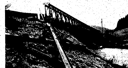
Third Bailey Bridge Across Our River at Auel
