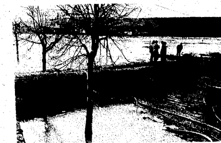
DIKES USED TO CONTROL HIGH WATER AT PONT-A-MOUSSON
