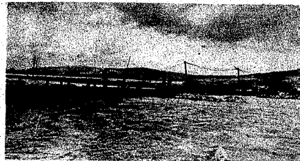
PONT-A-MOUSSON BRIDGE DURING HIGH WATER
