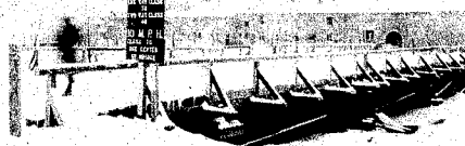
TIMBER TRESTLE BRIDGE AT DIEDENDORF OVER THE SAAR RIVER
