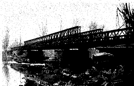
300-Foot Bailey Bridge Across Sure River at Bettendorf
