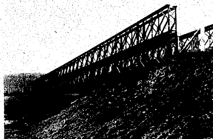
Bailey Bridge Across Our River at Auel
