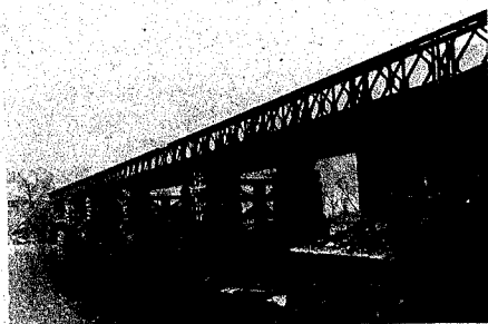
250-Foot Bailey Bridge Across Sure River at Wallendorf
