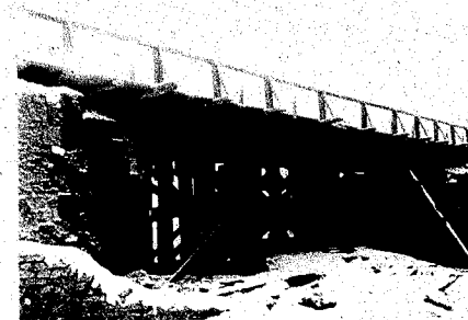
TIMBER TRESTLE BRIDGE OVER SAAR RIVER AT SAAR UNION
