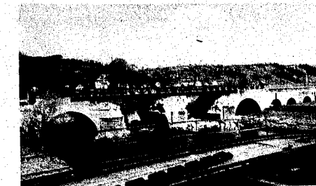
View of Bailey Bridge in Place at Kulmbach
