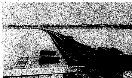
M-2 Treadway Bridge at Mainz - 1896 feet long; so far as known this was the longest tactical bridge ever built
