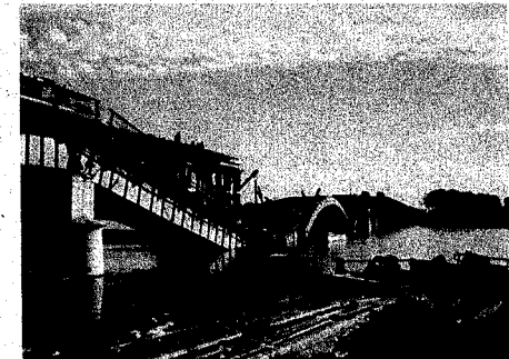
Bridge across Danube River at Deggenndorf under construction
