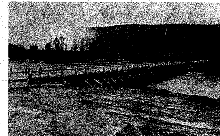
2-WAY PILE BRIDGE OVER THE MOSELLE AT ARNAVILLE (U-7647) SHOWING SMOKE SCREEN IN THE BACKGROUND
