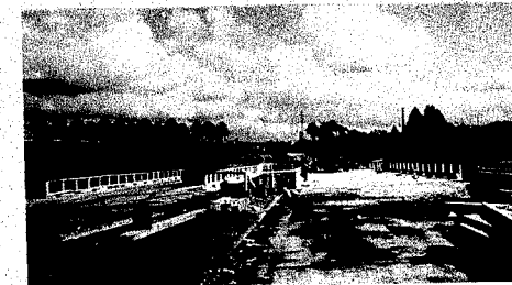
View of Autobahn Bridge East of Bayreuth showing Roadway of Completed Bridge
