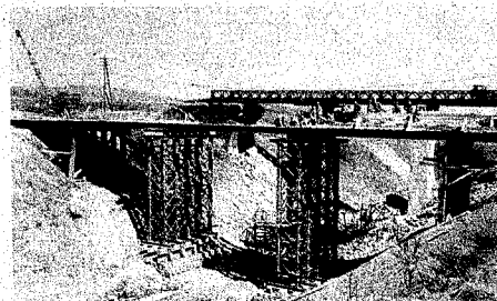
View of Overpass under Construction Using V-Trestle Piers near Waldrach
