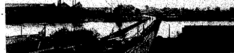
Heavy Ponton Bridge over the SEINE River at MONTEREAU. Length 400 ft. Built by the 88th Engineer Heavy Ponton Battalion on 25 August 1944.
