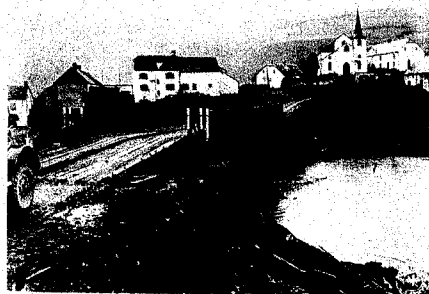
Bailey Bridge Across Our River at Eisenbach
