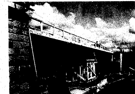
View of Autobahn Bridge East of Bayreuth Showing Bailey Bridge Panel Stringers
