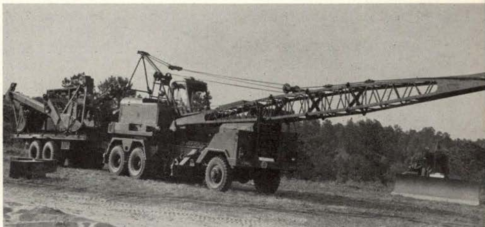
Even the crane used to erect a class 60 bridge is a behemoth. The 36-ton equipment-set eats two gallons of fuel per mile.
