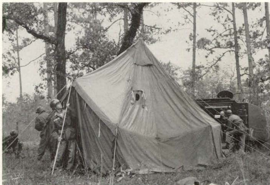
In five minutes erection is well under way.
