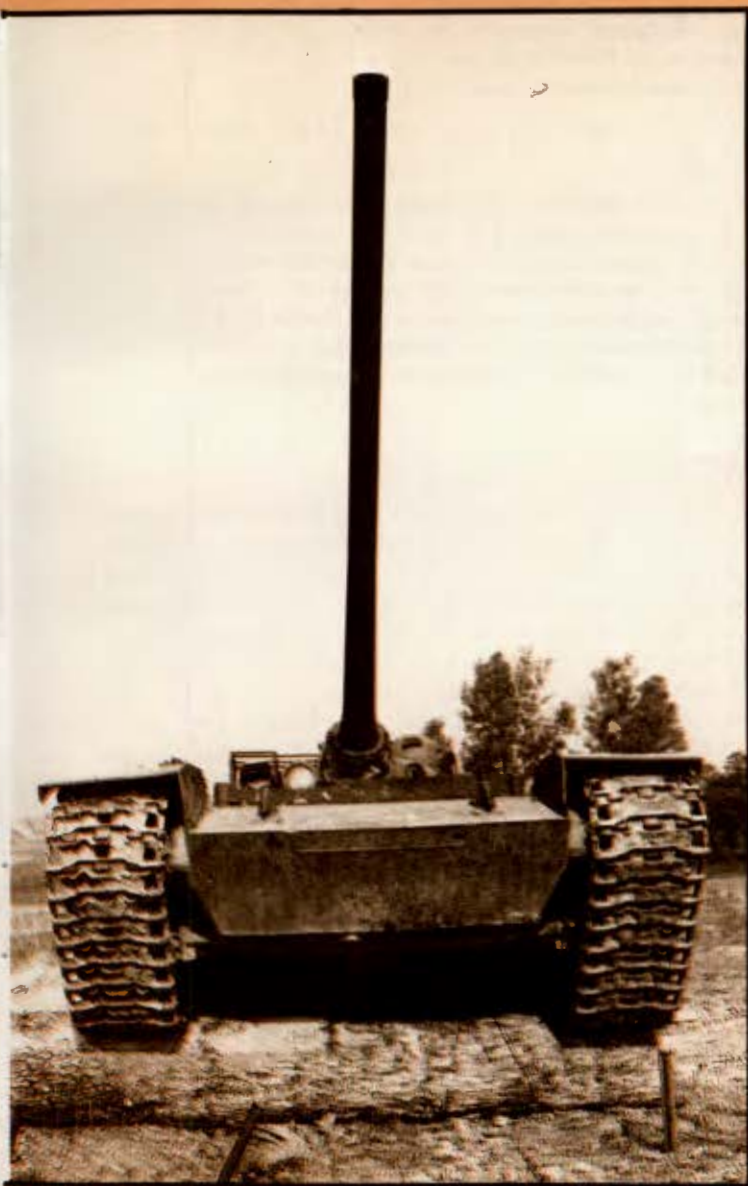
The tank shown here is a T-54 operated by a Patton Museum staff member. The tank was able to clear this particular hurdle, but it should be noted that the barrier was hastily constructed solely for the purpose of illustrating this article and was located on a lesser percent of slope than specified in the text. ED.
