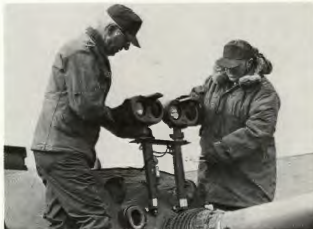
CW4 William Burkhardt (left) and SFC Edward Snook are shown mounting a Dover Device on a tank of the New Jersey National Guard.
