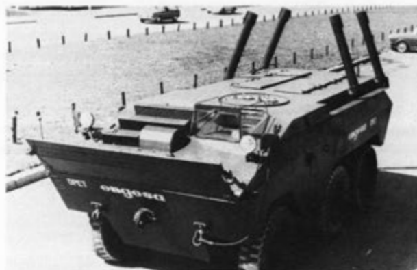
Capable of transporting 15 men over land and water, the CTRA is a 23,500-pound steel-armored vehicle. Two versions are now in production: a Marine model with shrouded propellers and steering vanes; and a model for use by the Army without the water propulsion equipment.
