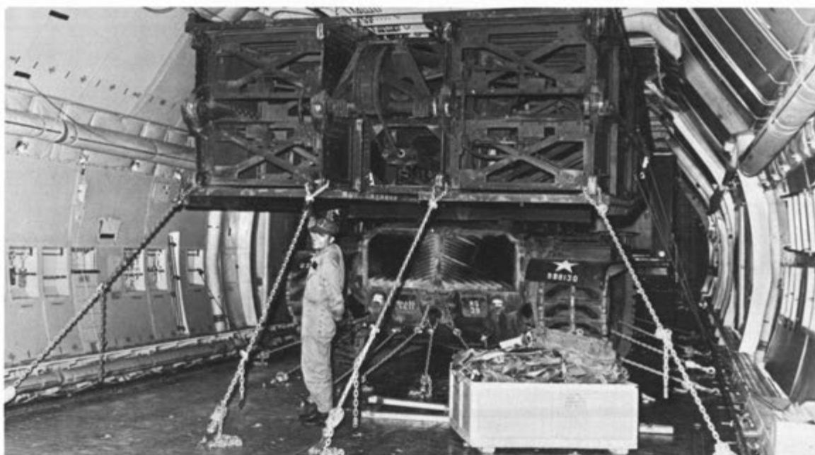
During recent tests the 121,000 AVLB was flown from Pope AFB/Ft. Bragg to the Lockheed plant at Marietta, Ga. Even with the 40-foot scissors bridge aboard there was plenty of room to accommodate the additional 67,000lbs of cargo which could be carried.
