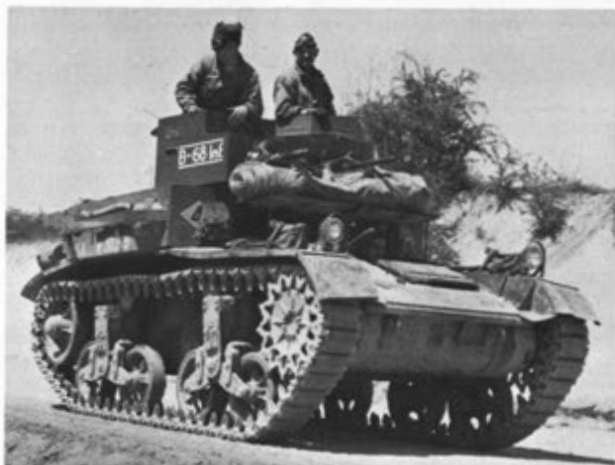
M2A3 light tank of the 68th Infantry at Fort Benning in 1940. The M2A3 appeared in 1938. Maximum armor was .75 inches and weight was 13 tons. Speed was 40 mph. Armament consisted of a .50 caliber machinegun in one turret and a .30 caliber in the other.
