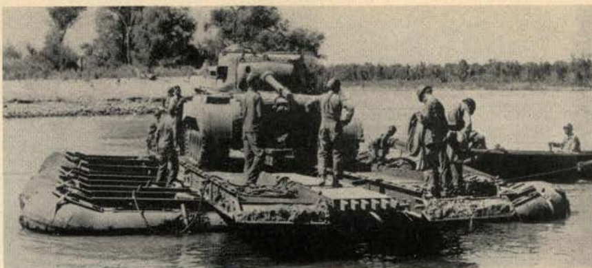
The four-float raft ferrying a 35-ton tank.
