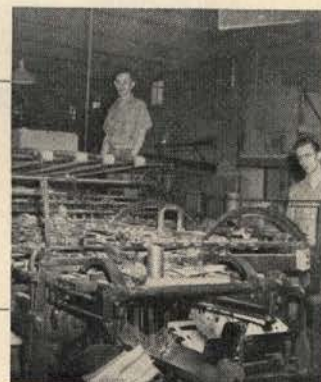
Printed sheets must be folded and folder operators Pyles (upper) and Robins quickly put them through this Dexter folder in 32-page signatures (16 pages on each side of the sheet).
