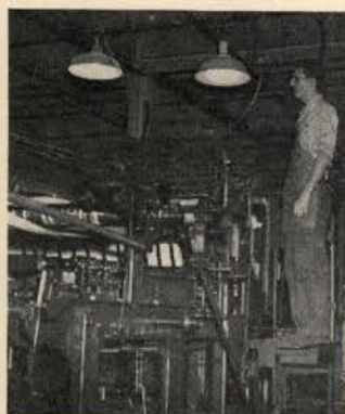
Big, automatic-fed Miehle presses like this one in charge of pressman Thomas are made ready in 16-page forms and the sheets of the magazine begin to roll off.
