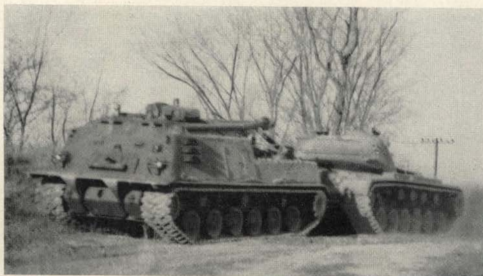
The T88 Assault Recovery Vehicle, Medium, is shown towing an M48. It is using the main winch which has a capacity of around 90,000 lbs.
