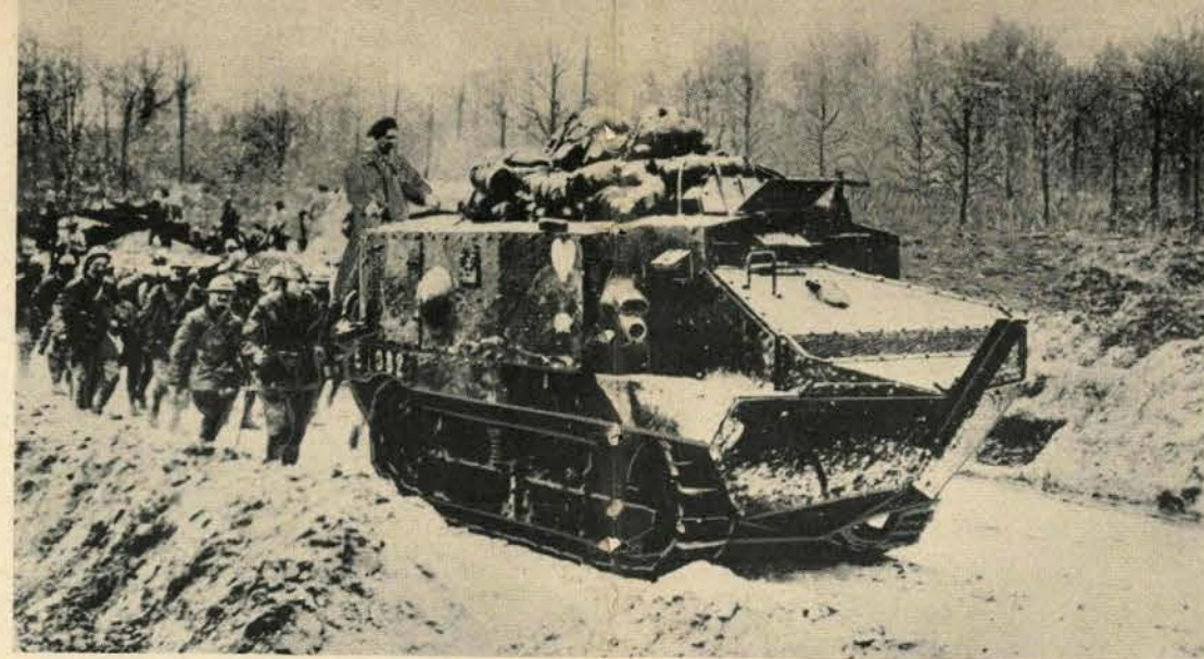
The French Schneider in action. It carried a 75mm cannon and had an amazing speed of 4 mph.
