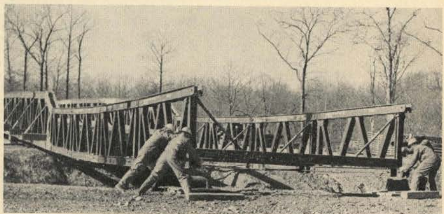
The T-6 bridge reaches the far end of the gap after being pushed into position by a bulldozer.
