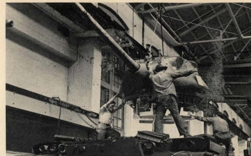
The turret goes on an M47. The gun is operated by two separate electric hydraulic fire control systems. Tank commander or gunner can operate the weapon.
