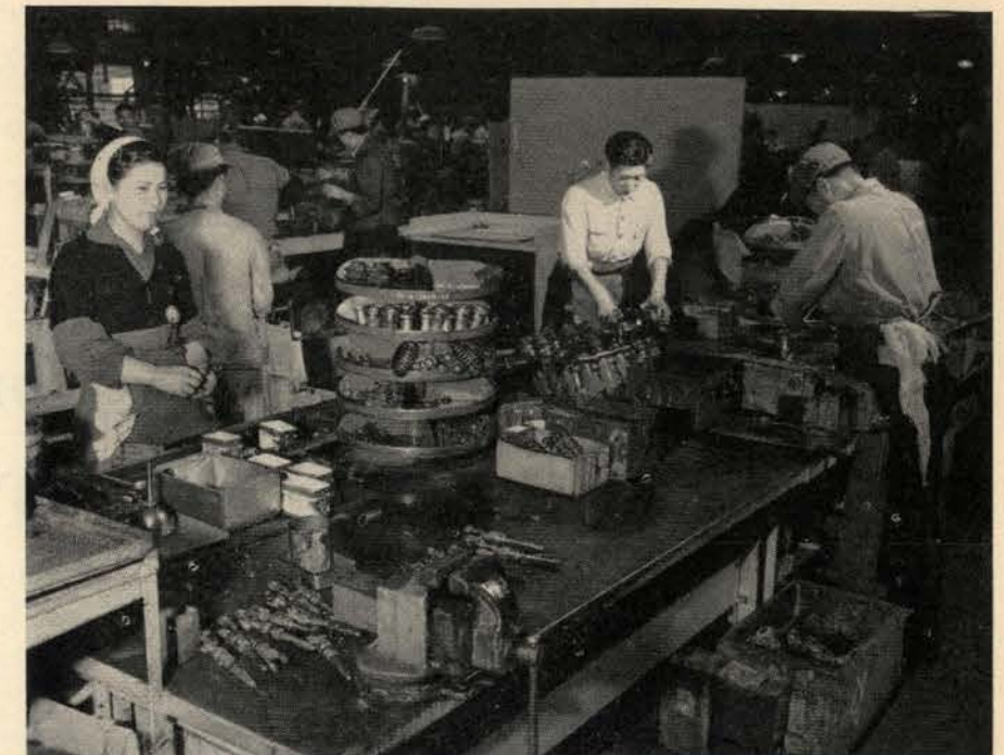
Small assemblies are broken down and component parts segregated into their proper bins. After cleaning and rebuild they will be reassembled by the workers.
