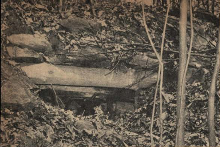
Demonstrating Japanese defensive tactics will call for a good deal of digging-in. Bunker shown is 8 feet by 6; is constructed of native material, and has a low firing port.
