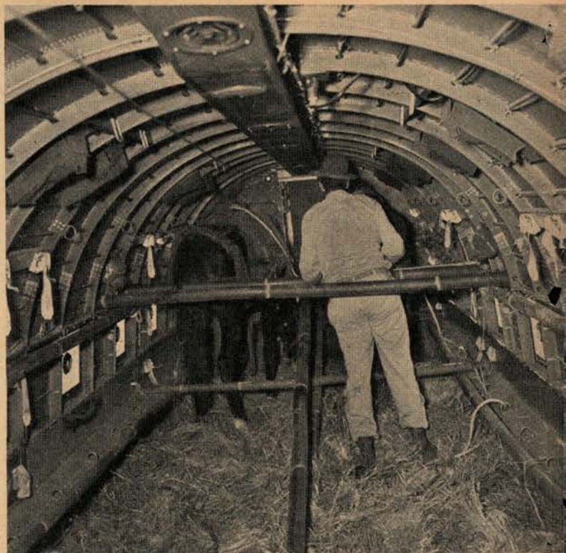
Stalls for airborne animals in C47s were constructed, as seen in this photo, from bamboo poles. Two animals have already been loaded. Note hay on floor for secure footing.
