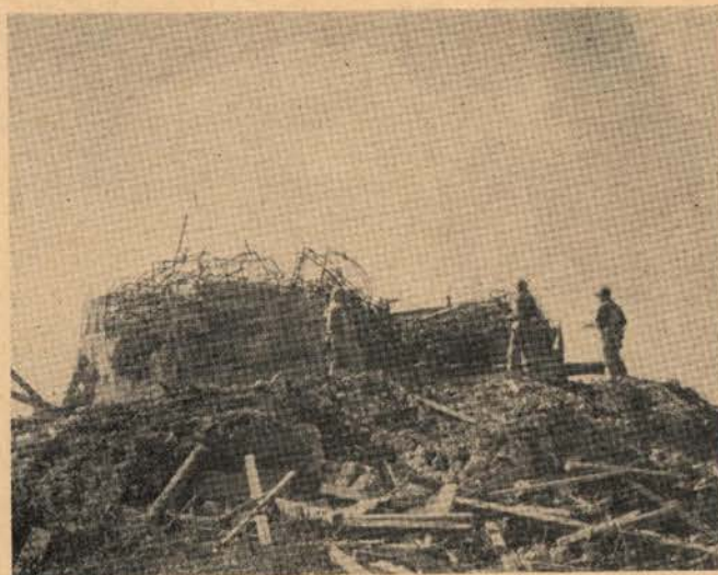
This large reinforced concrete pillbox housed a 6-inch gun, and proved a tough, strong point to break. Defense points were placed to make possible mutual fire support.
