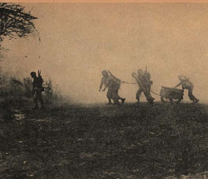
Chemical Warfare troops trundle the 4.2 chemical mortar through a smoke screen. Mortar, which has been nicknamed the "goon gun," can fire 20 rounds a minute up to two and one-half miles; fires either smoke or explosives.
