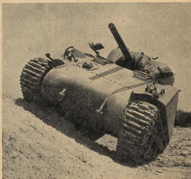
Fig. 3.—This guy defied the law of gravity—but he broke his rear idler housing doing it.
