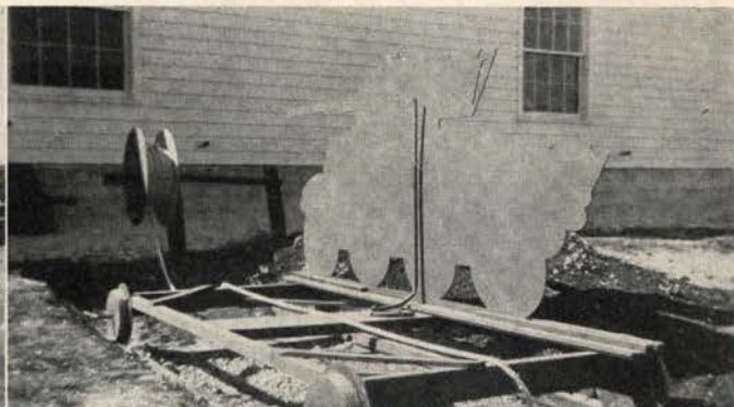
A windlass and an operator are employed at each so that the silhouettes can be moved in either direction on the track.
