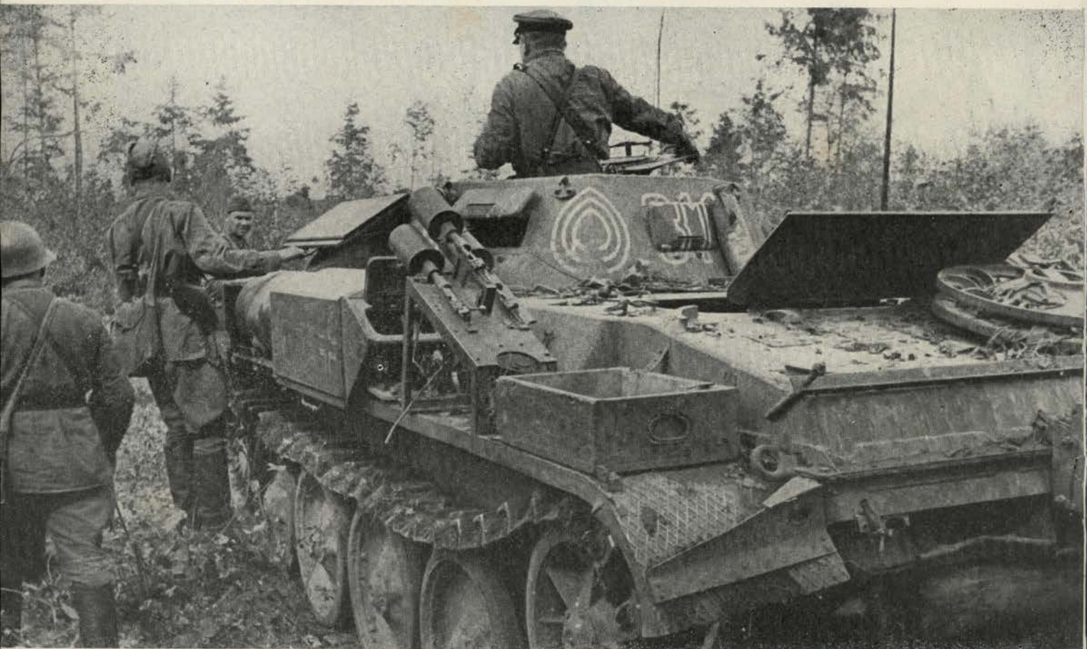
The captured nine-ton Mark II tank pictured above, is on its way to a Russian salvage depot. It has two independent flame-throwers, one mounted on each front track-guard. Of short range, these flame-throwers are effective only against personnel.
