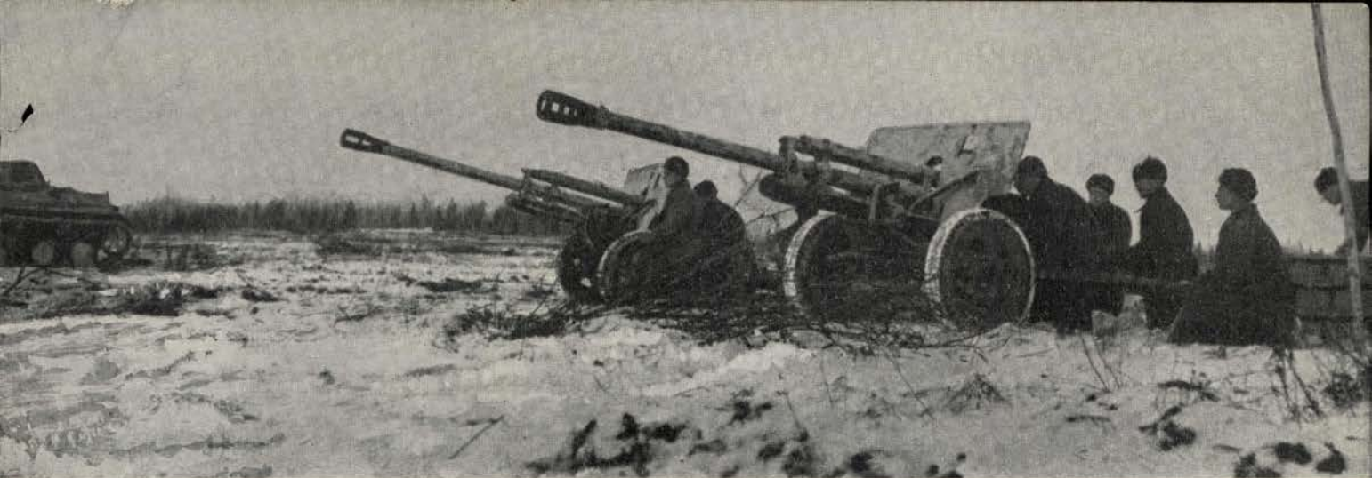
The 57mm AT guns in action, showing muzzle brakes very like the German 50mm.
