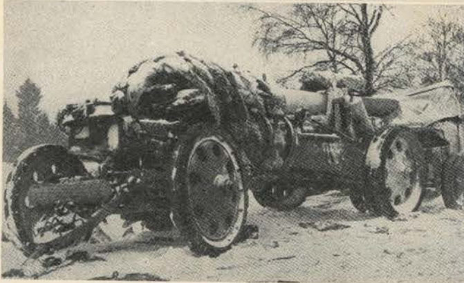
This damaged 210mm howitzer, discarded on the Kirov highway by the retreating Germans, has a range of more than 10 miles and fires a 264 pound shell. It is part of the German GHQ artillery.
