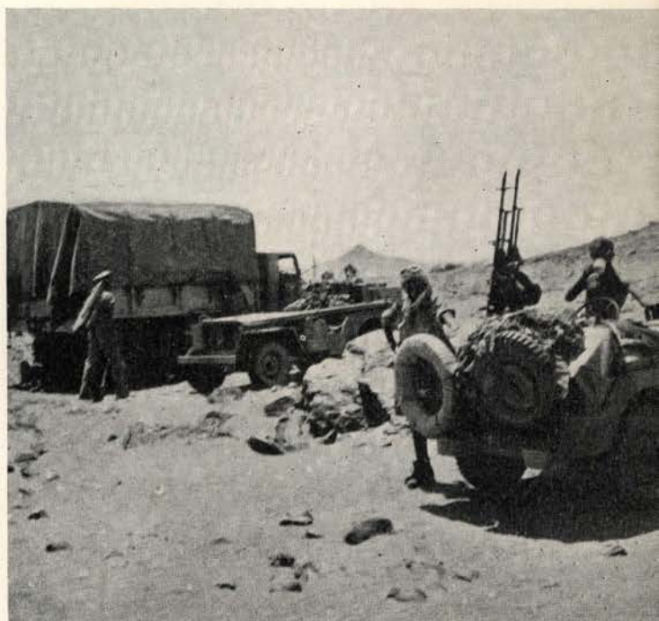
Two jeeps and a truck of Captain Smith's party break camp the night before the Bengasi raid. Each jeep mounts four .30 caliber machine guns in pairs, which can be shot either simultaneously or individually. Note the two sets on jeep in foreground.
