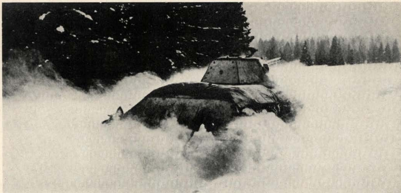
"With special equipment like widened tracks and grousers, tanks can negotiate snowfalls of three and four feet, and sometimes more."
