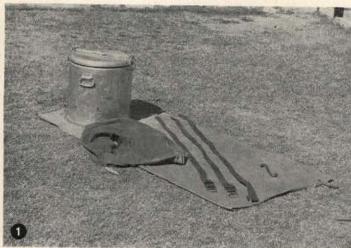
1—One unit of the hoot-food-container carrier. 2—The carrier from above. Note the "S" hooks and the lateral support given by the straps. The cover was made by the troop saddler out of salvage tentage.
