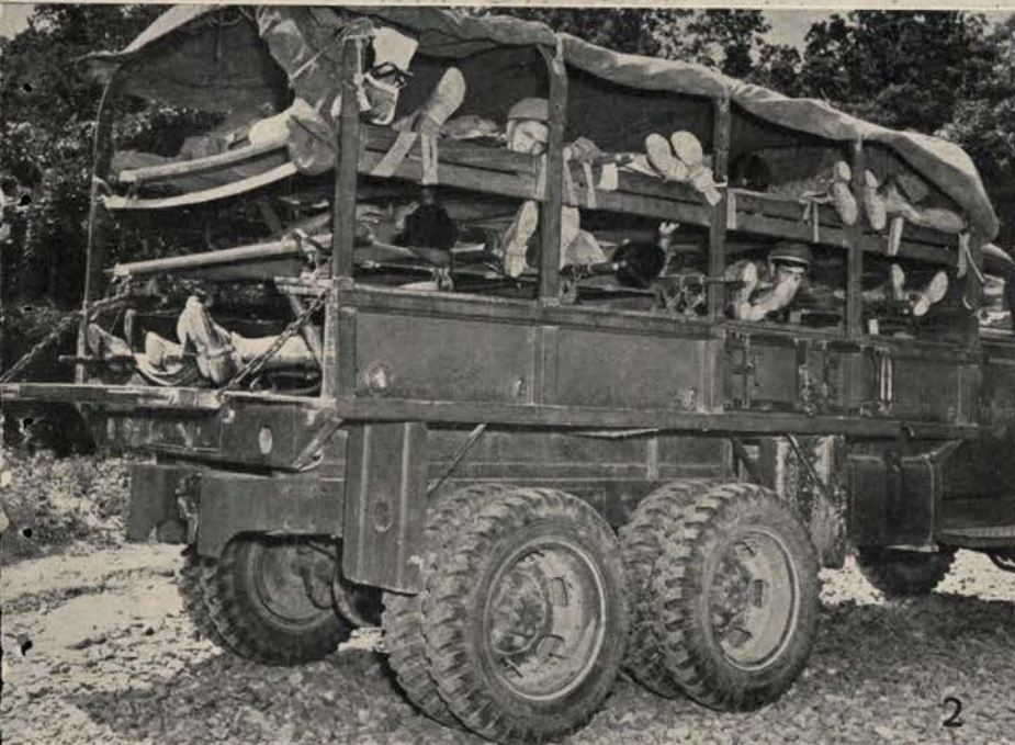
1—Rear view of surgical truck (experimental) 47th Medical Battalion (Armored) in operation. 2—Side view of 2½-ton cargo truck loaded with 15 litter patients. 3—Surgical team in truck.
