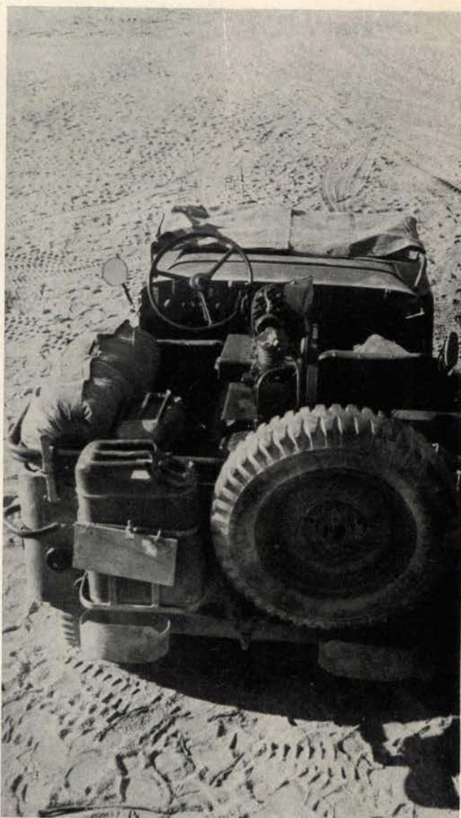
The air compressor mounted on a jeep was the antidote for cactus punctures.
