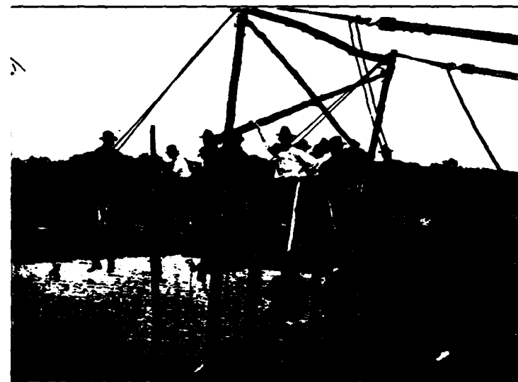
REES' PILE BRIDGE. SETTING PILES.
