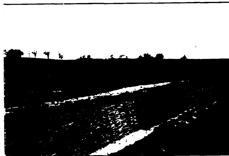
CONTINUOUS HURDLE, SOD AND FASCINE REVETMENT.
