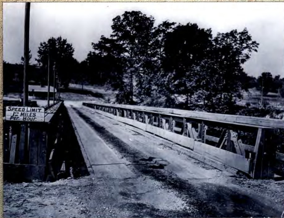
Upatoi Creek Bridge, after the Pershing Floods, c. 1923.
