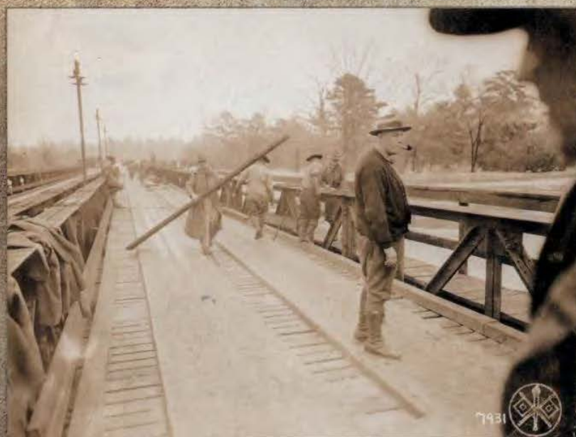
Finishing construction on the Upatoi Creek bridge, January, 1923.
