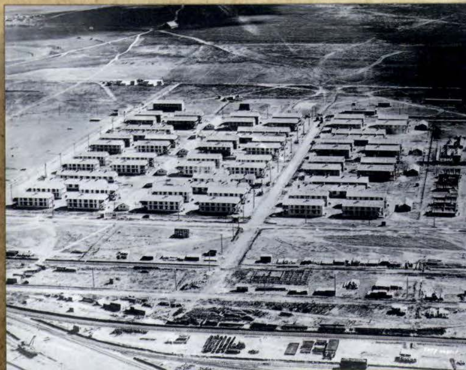
Camp Benning, erected within the first 6 months of Camp Benning's transition to the Main Post location, June, 1919. These two-story wooden structures, railroad system, power lines and telephone lines helped establish the permanency of the post.
