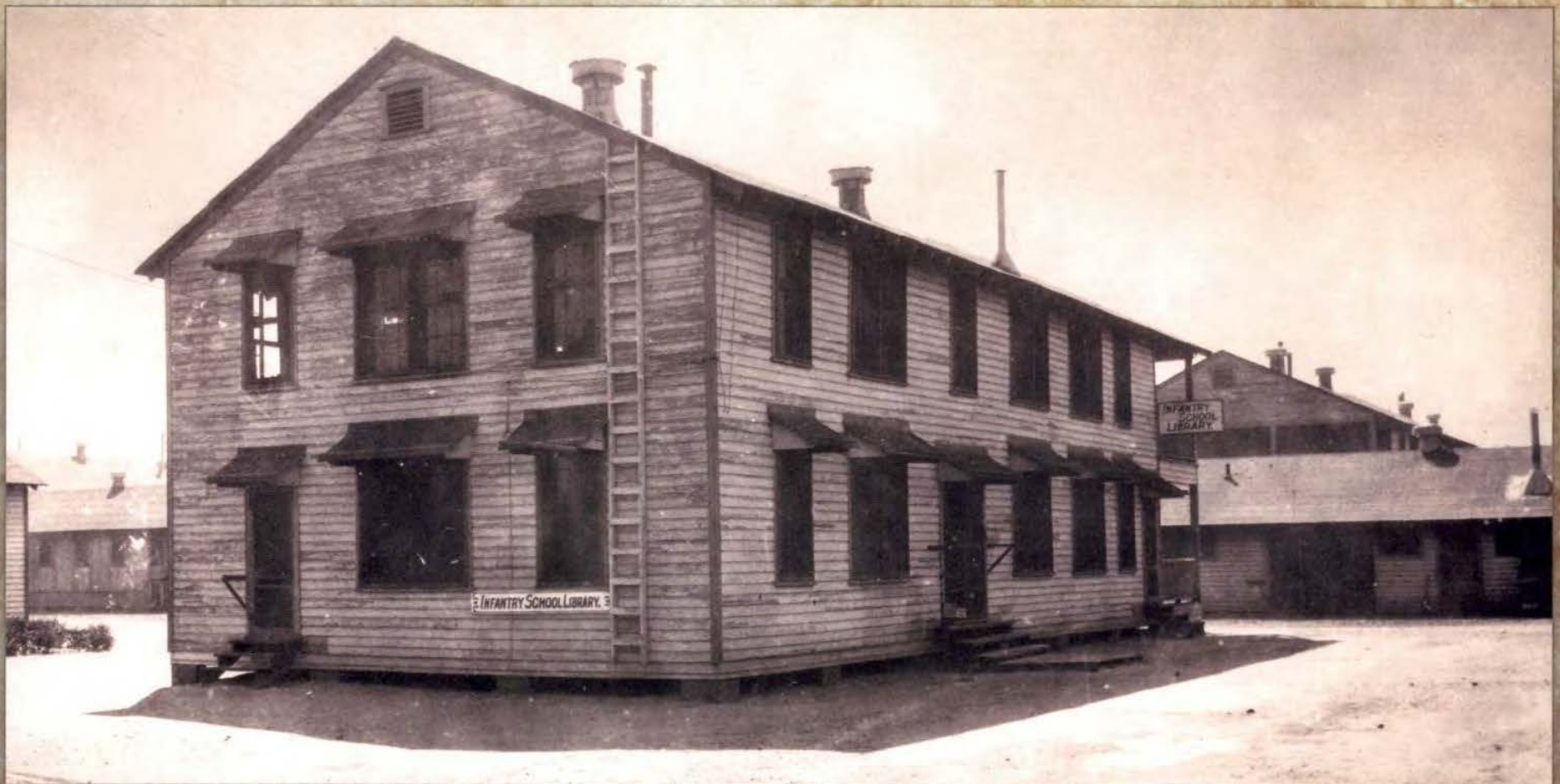
The Infantry School Library, 1925. This building housed the Infantry School Library until it was moved into the Infantry School building on August 7, 1928.
