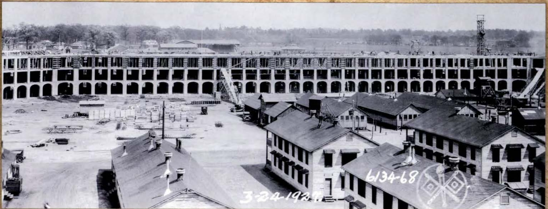
29th Infantry Barracks, March 24, 1927. On February 6, 1925, construction began on the 29th Infantry Barracks, the 1st of 3 large square groupings of buildings with central courtyards known as the "Cuartels," which is a Spanish word meaning "barracks."
