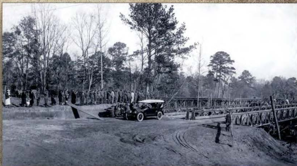
Upatoi Creek Bridge, 1925.
