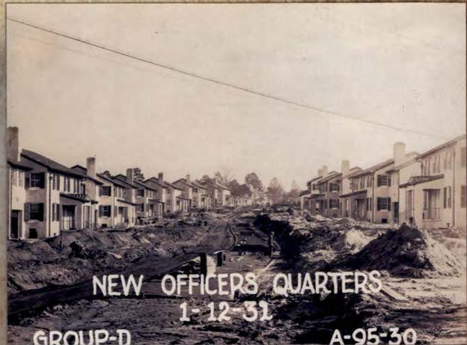
New officers quarters, January 12, 1931. The 1930s was marked not only with the Great Depression, but with large government construction projects to help simulate the economy.
