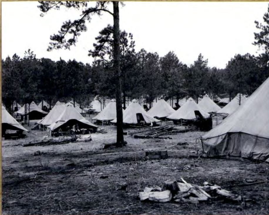
By the end of the 1930s the world situation was more ominous. As part of mobilization preparations, units of the 1st Engineers arrived in October, 1939 to clear ground for the first contingent of the 1st Infantry Division and by November, 1939 the entire Division occupied a "tent city" near Kissick Pond.
