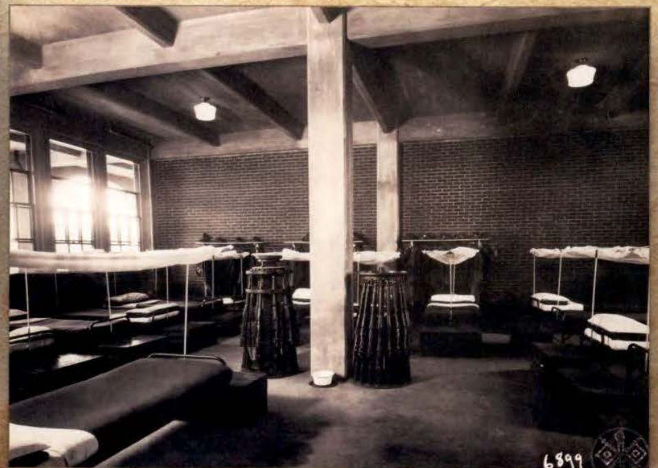
View of the new barracks interior, c. 1929, which constituted a great improvement from the wooden structures and tents the 29th Infantry previously inhabited.
