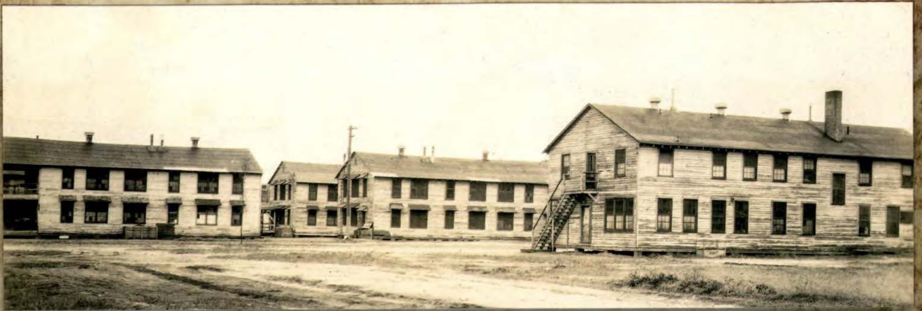
The first Infantry School of Arms was completed on October 26, 1918. On February 22, 1919, 100 West Point graduates became the first class to finish the course while the school was at the Macon Road location. Pictured above are the two-story wooden structures of the new camp that comprised the academic area on what is now Stillwell Field, c. 1920s.
