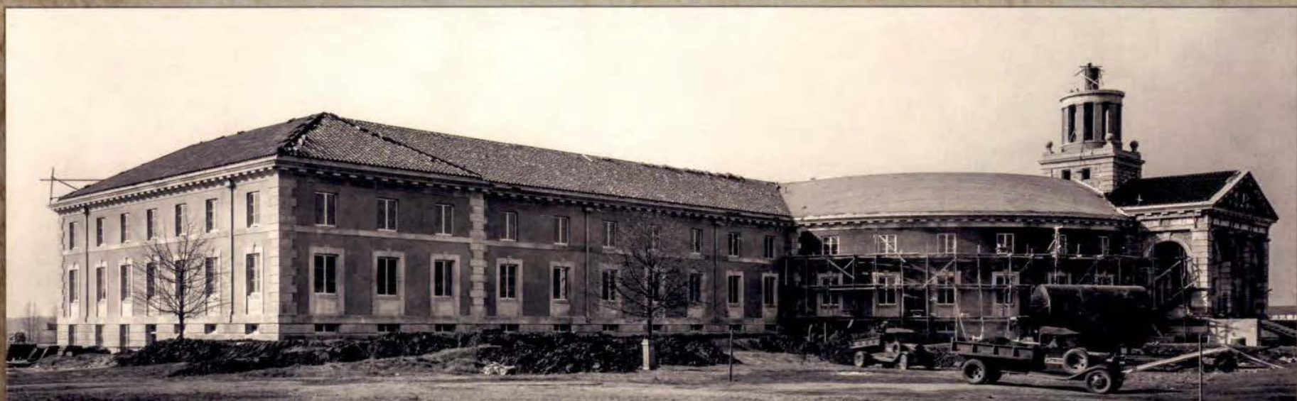
Front view of The Infantry School, 1935. Built with a design of stately grandeur, The Infantry School served in its role as head of infantry training and Post Headquarters until 1964, when Infantry Hall (Building 4) was completed.
