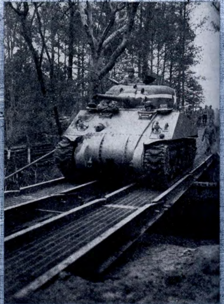
An M4 Sherman Tank weighing 30 tons crosses a ravine using a steel trestleway constructed by the 55th Engineers, Fort Benning, 1943.
