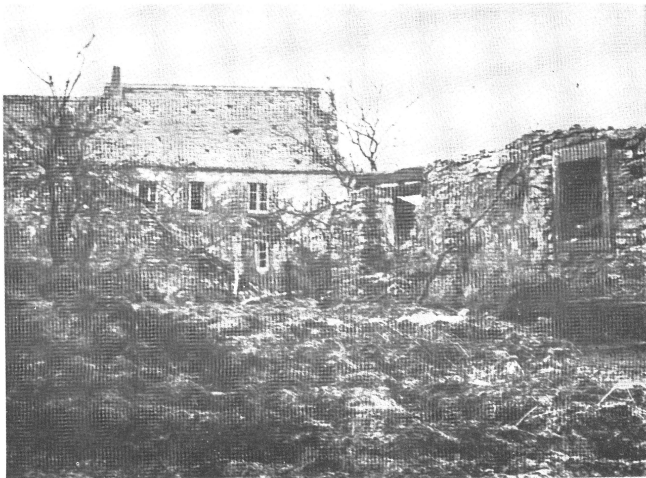
COURTYARD and manure pile for Houses 8, 9, and 10, where Lt. Cook parked his tank. View north. Note heavy stone construction.
