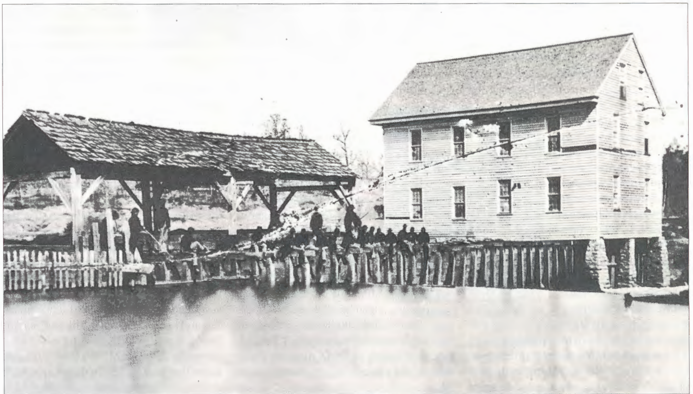
Lee and Gordon's Mills on West Chickamauga Creek. It served as a grist mill and a saw mill.
